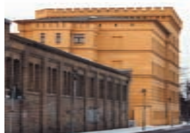
Riding arena by Schinkel, Potsdam, Schiffbauerdamm 2000 m 2 interior wood panellings treated with SAICOS COLOR WAX finish by Painters Knauff Ltd., Nauen, Mr. Knauff, tel. 03321/453809
