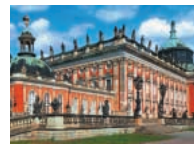
Neues Palais (New Palace), Potsdam/Park Sanssouci, 500 windows treated with SAICOS HOUSE & GARDEN-COLOUR (WINDOW & DOOR-PAINT) by Geltower Holzwürmer, Geltow, Mr. Grünberg, tel. 03327/55578
