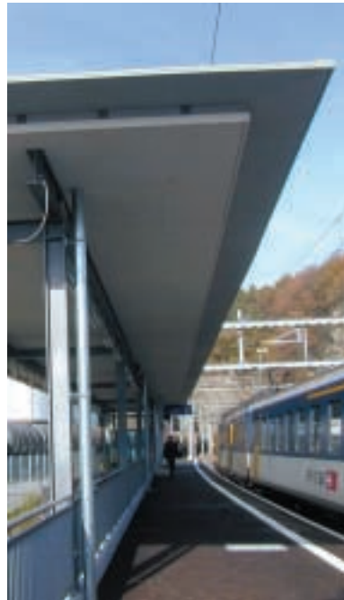
Roofs on more than 100 railway stations all over Switzerland, here: railway station Männedorf on Lake Zürich Balteschwiler wood pretreated with SAICOS BEL AIR white and agate grey
